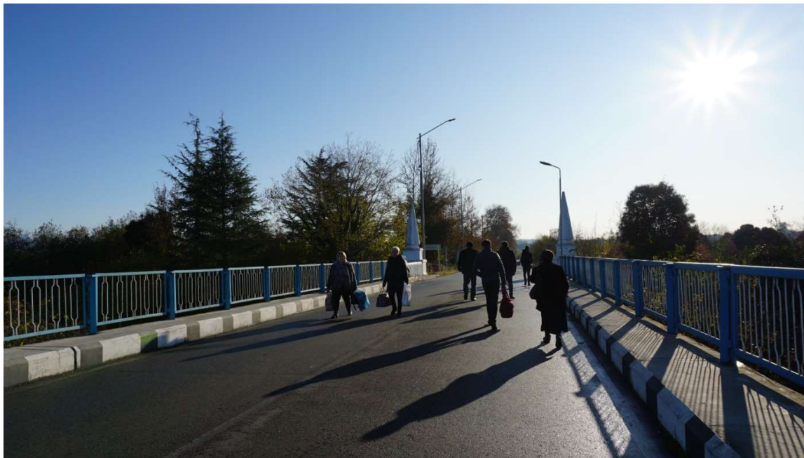
Enguri Bridge. Citizens moving to the Georgian-controlled territory. November 22, 2019, first half of the day
